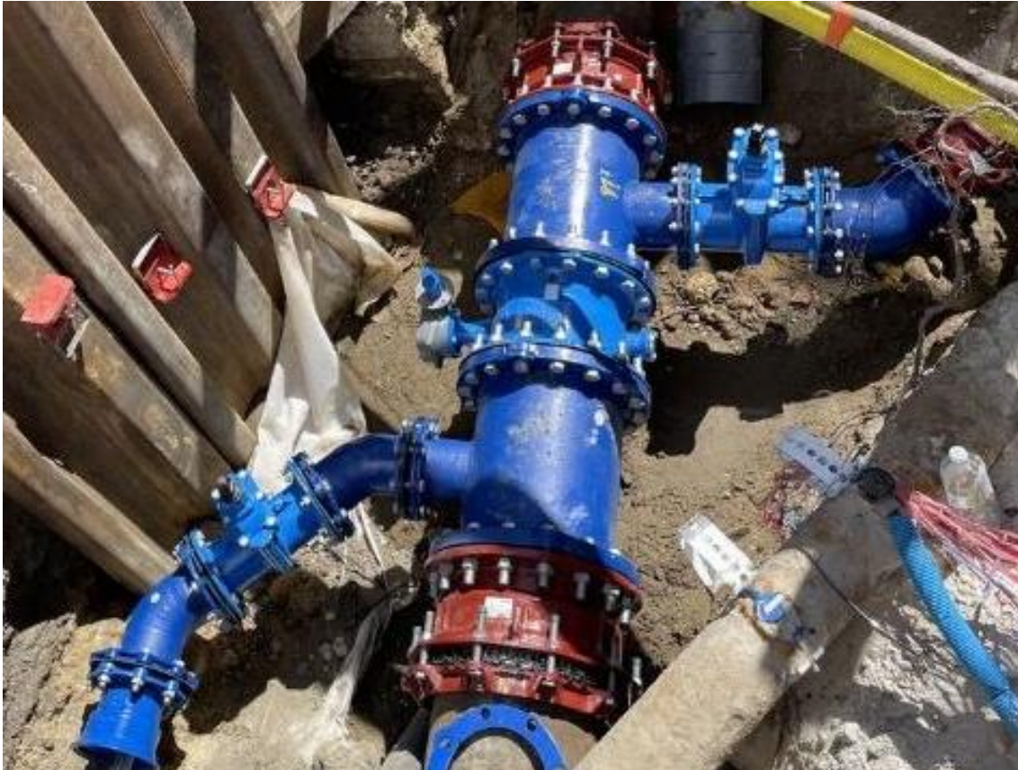
GF MultiJoint and VAG flanged double offset butterfly valve in Tuscany (IT)
