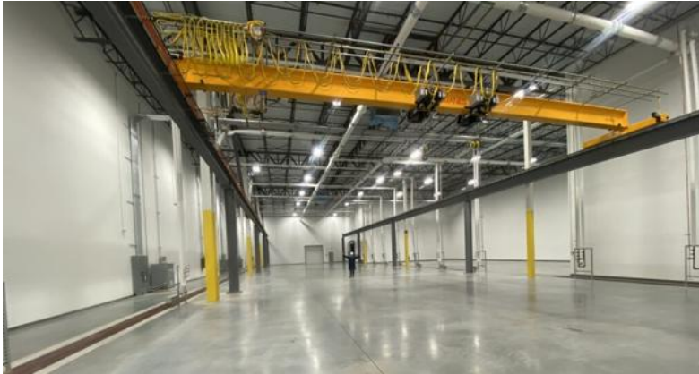
Atlanta site, before ramp up
